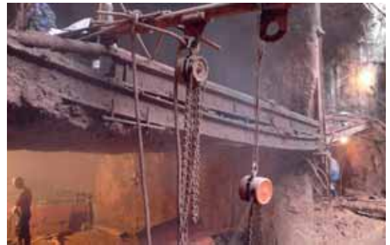
Jinsha Zhou Tunnel, CRD Vortrieb; Wuhan – Guangzhou PDL, DK 2196,3
