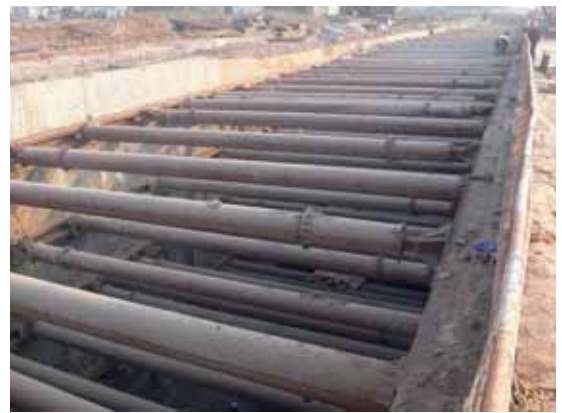
Jinsha Zhou Tunnel, offene Bauweise; Wuhan – Guangzhou PDL, DK 2196,5
